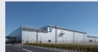
Ishihama Plant Address: Higashiura-cho, Chita-gun, Aichi Products: On-board batteries
